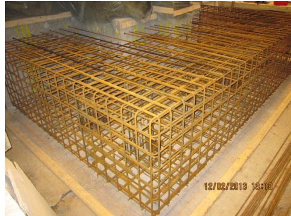
Figure 20: Reinforcement of the foundation extension.
